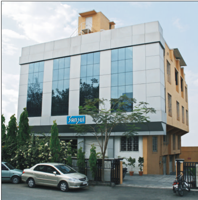
Automatic Calibration facility for Loadcells.
